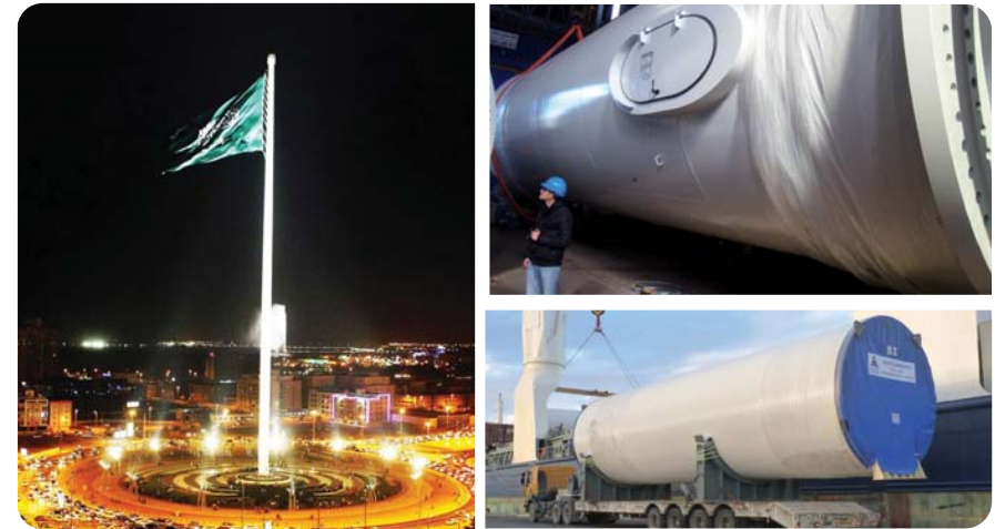
Project: Supply and Fabrication of The tallest flagpole in the world (H:170 m, Diam from 2,3 m to 4 m) located at Jeddah, KSA Client: Al Babtain-Le Blanc Owner: Abdul Latif Jameel (Saoudia Arabia) Year: 2013 / 2014
