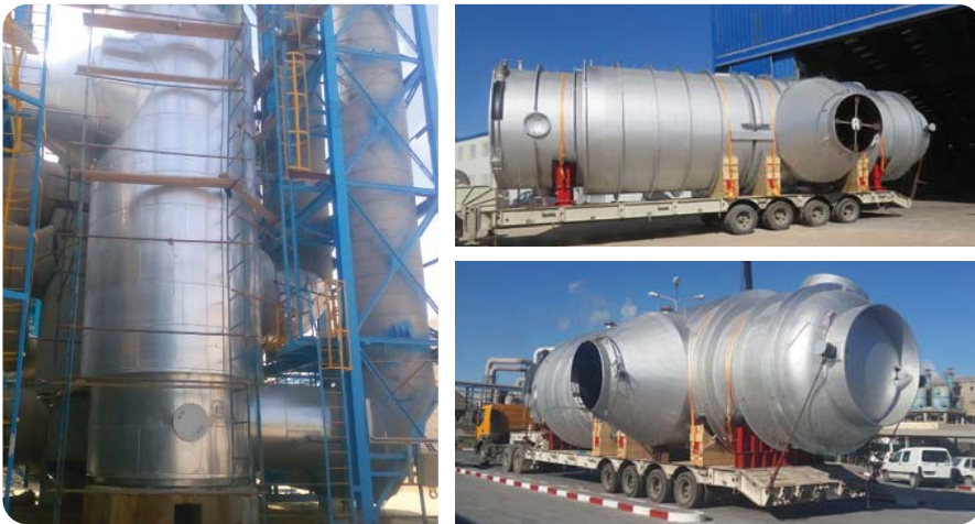
Project: Retubing with replacement for calenderer and tube sheets of two gas exchangers gas SG 3504 A /B for the DAP plant in Gabes Owner: GCT Groupe Chimique Tunisien ( Tunisia) Year: 2014
