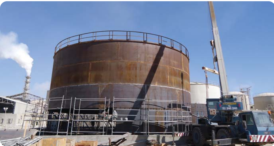
Project: Construction of a sulfuric acid storage tank with a capacity of 6500 T Owner: GCT Groupe Chimique Tunisien ( Tunisia) Year: 2012
