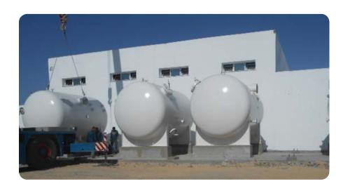
**Project:** Design , Supply ,Fabrication & delivery of 10 sand filters for Brackish Water Desalination plants : Kebeli , Souk Lahad & Douz
