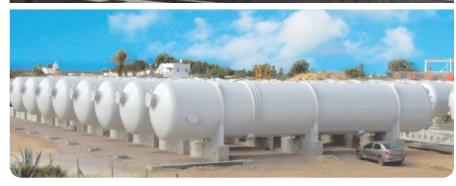
**Project:** Design, Supply, Fabrication, Delivery & Construction of 14 sand filters (L:24m; Ø: 4m) For Djerba Seawater Desalination Plant
